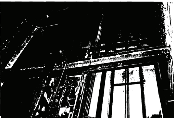
Figure 8. Damage state 9: in the Northridge Hospital Medical Center, 1967 Westinghouse elevators 1-4 all experienced damaged car rail brackets. Here, the spreader beam running horizontally through the photo is bent. The car rail guide running vertically through the photo in the left 1/3rd is attached to the beam and is bent with it. Repair was carried out by inserting shims between the bent spreader beam and the car rail bracket.
